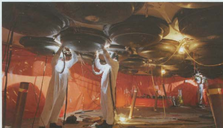
Decommissioning work at Hunterston A
