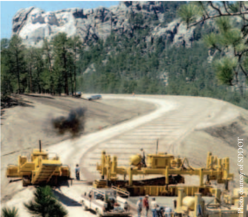
Paving concrete on the recently completed highway to Mt. Rushmore.
